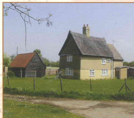
No.59 High Road - the only thatched vernacular cottage in the conservation area
