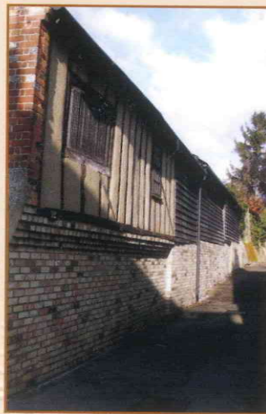
Curtilage listed building at no.52 Church Street
